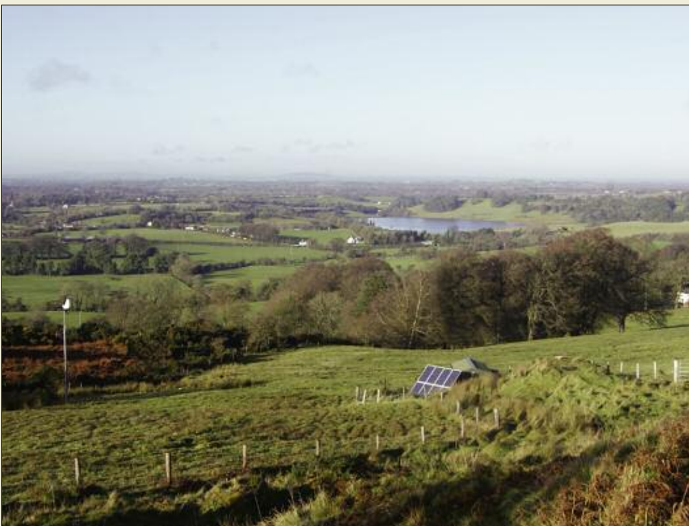
Wind and solar energy provide the electricity required to run the drinking water treatment plant at Blakestown/Brittonstown in County Wicklow.
