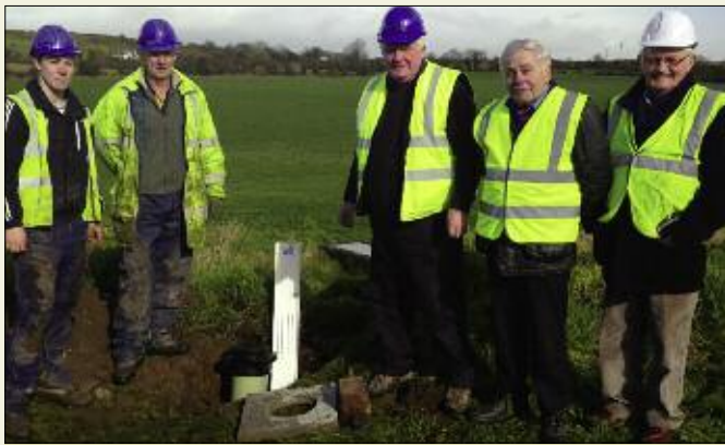
Replacing meters on non domestic connections on Lough Gur GWS.
